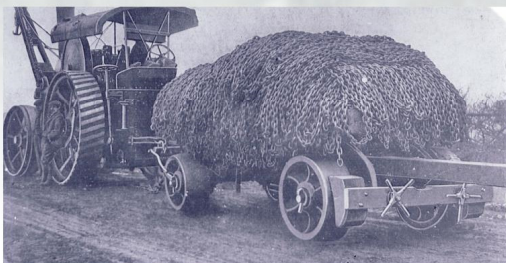
One MINE CHAIN , 1 1/2 inch diameter, length 3220 yards, weight 2 1/2 tons, 13 cwt. 1 qr. 0 lbs. The Carriers, (L. & N. W. Joly Cox) state that this is the longest and heaviest chain in any length despatched from the Black Country for many years. Makers—ELIZA TINSLEY & Co., OLD HILL, Staffs.
